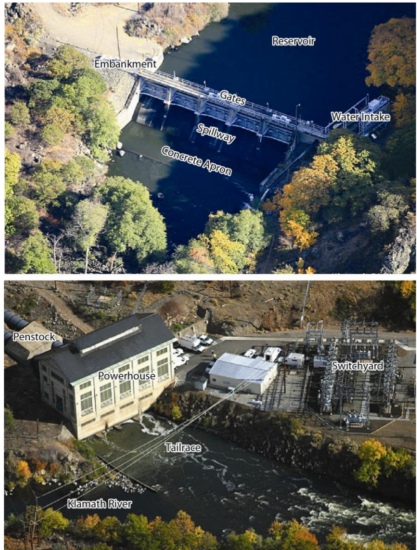
Figure 4.2-8: Photo of Copco 2 Dam and Reservoir with Specific Components Labeled. With full facilities removal, all visible components would be removed. With partial facilities removal, certain components (e.g., penstock) would be retained.
