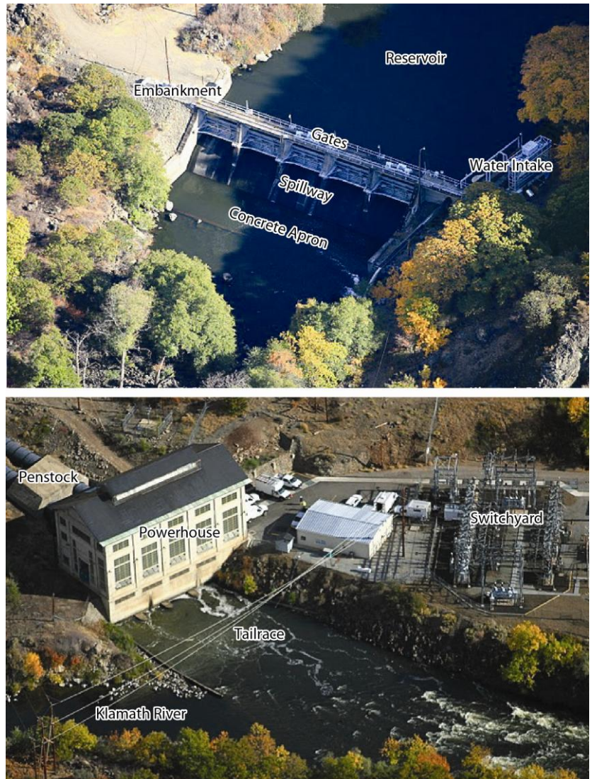
Figure 4.2-8: Photo of Copco 2 Dam and Reservoir with Specific Components Labeled. With full facilities removal, all visible components would be removed. With partial facilities removal, certain components (e.g., penstock) would be retained.
